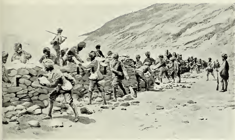
DISMANTLING LOOP-HOLED WALL AT KANGMAR
